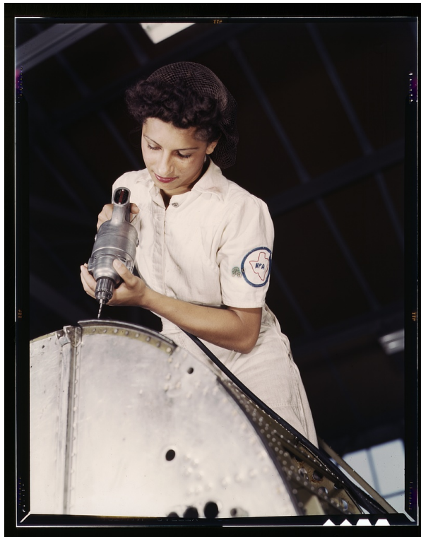
Fig. 9. Howard R. Hollem, Oyida Peaks riveting as part of her NYA training to become a mechanic in the Assembly and Repair Department at the Naval Air Base, Corpus Christi, Texas, août 1942 ©Library of Congress
